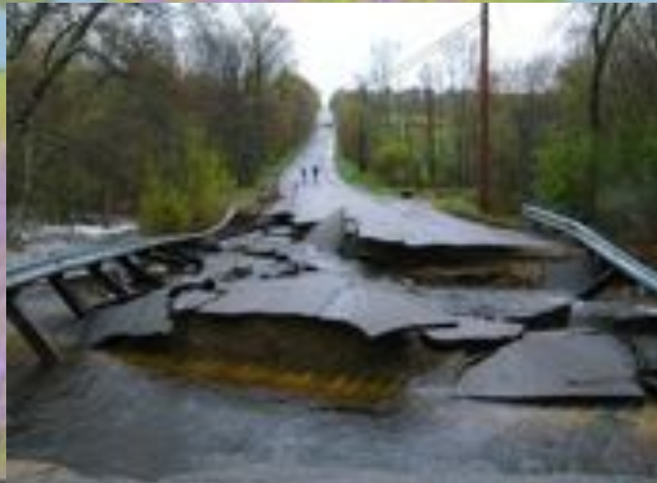
Bridge over Axe Handle Brook, Rochester, NH May 2006.
